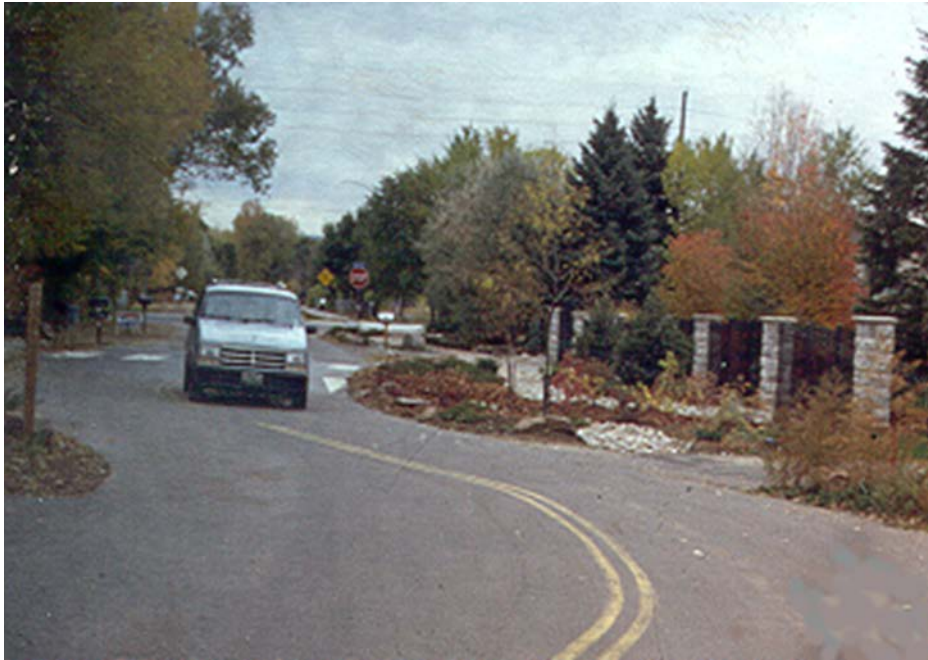
Poorly designed chicane
