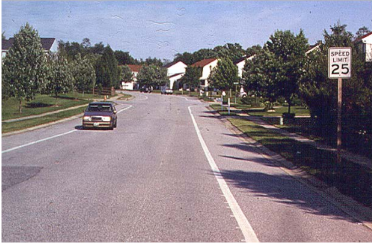
Markings to Narrow Lanes
